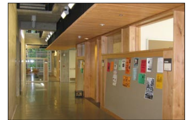
Interior circulation corridor receives direct daylight from window at end of hallway and borrowed light from transom window above internal partition wall of classroom.
