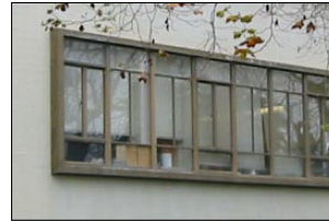
Raised frame window surrounds, suited for north and east building facades
