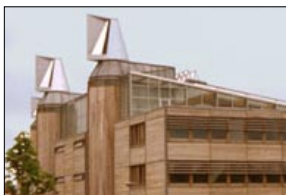
Tracking windvanes atop stair cores ensure that natural suction creates a thermal chimney effect, exhausting warmed air on this classroom building at the University of Nottingham's Jubilee Campus.
