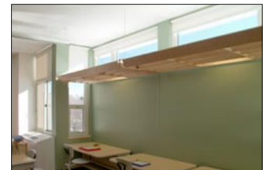
Interior light shelves facilitate deep daylight penetration without glare.
