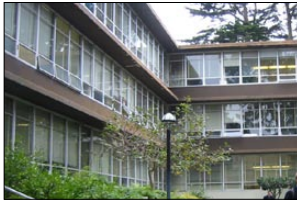
Continuous horizontal sunshading above horizontal ribbon windows, on facades facing south and west
