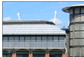
Continuous ridge vents along the shallow-pitched roof of this office building at the Inland Revenue Centre in Nottingham. The glass cylinder stair tower has a fabric roof that lifts to allow the escape of exhaust air.
