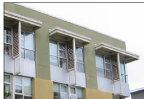
Operable windows and external shading devices on the Student Services building
