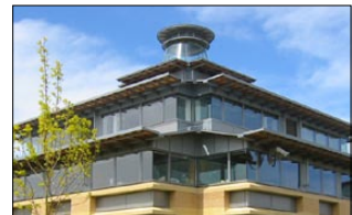
Thermal chimney atop a new research facility at the Centre for Mathematical Sciences, Cambridge University
