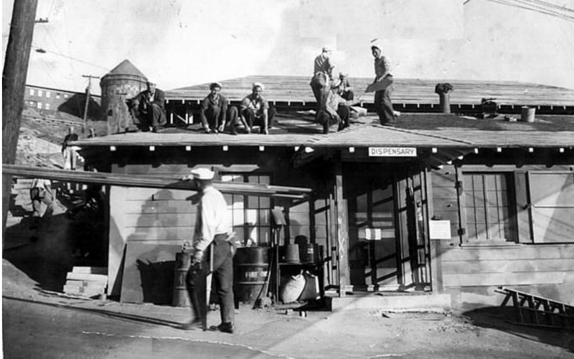
Figure 80: Building 37 (Dispensary) being roofed (ca.1942-43). Source: RTC Archives.
